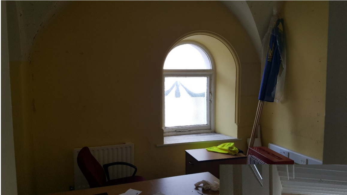
<- Typical arched window in vaulted room
