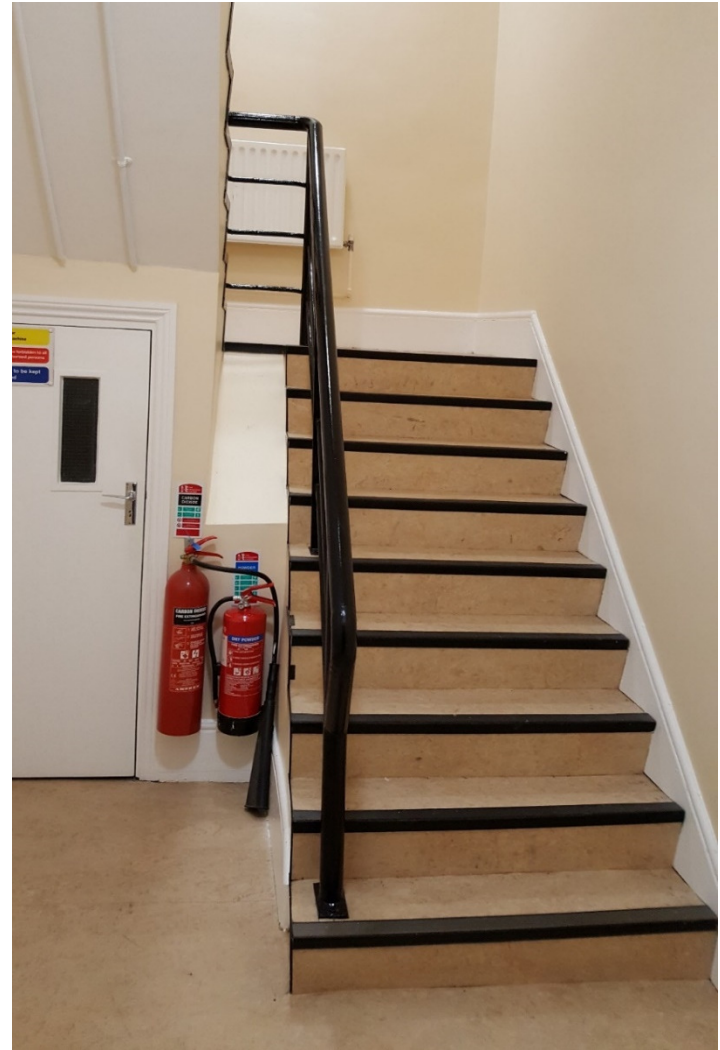
Existing central concrete stairs to be removed, to be replaced with new stairs to comply with Building Regulations
