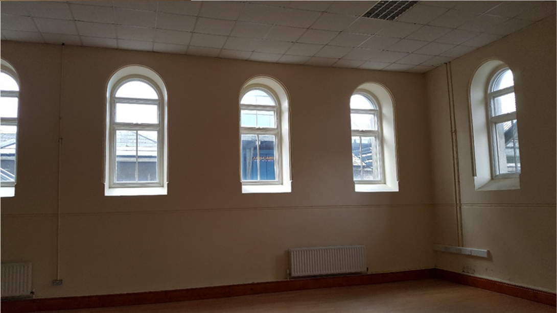
Existing windows to be removed and arched openings to new adjoining library space to be formed
